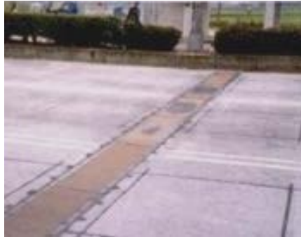
Figure 5.3 – Typical WIM station coupled with double loop detectors (taken from wim.zag.si ).
