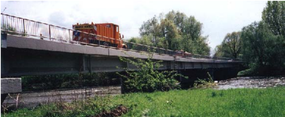
Figure H1. Mura River Bridge
