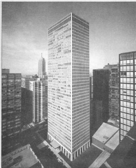
Constructed in 1964, Chestnut-DeWitt Apartments was the first tall building to employ the framed tube structural system. (Photograph by Hadrich-Blesing, courtesy of Skidmore, Owings & Merrill LLP)
