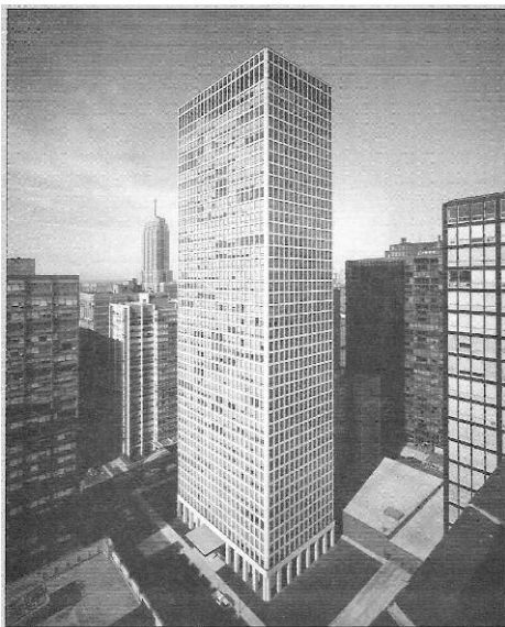
Constructed in 1964, Chestnut-DeWitt Apartments was the first tall building to employ the framed tube structural system. (Photograph by Hadrich-Blesing, courtesy of Skidmore, Owings & Merrill LLP)
