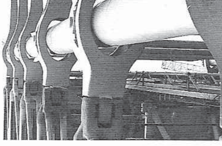
Gerberettes punctuate column. Space between gerberette and column lightens and articulates connection.
