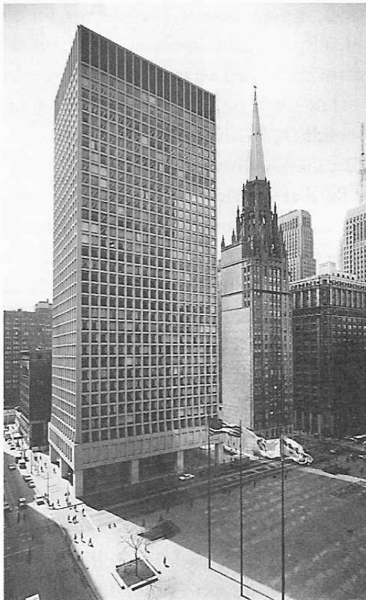
Brunswick Building, completed in 1965. The Chicago Civic Center Plaza is seen in the foreground. (Photograph by Hedrich-Blessing, courtesy of Skidmore, Owings & Merrill LLP.)
