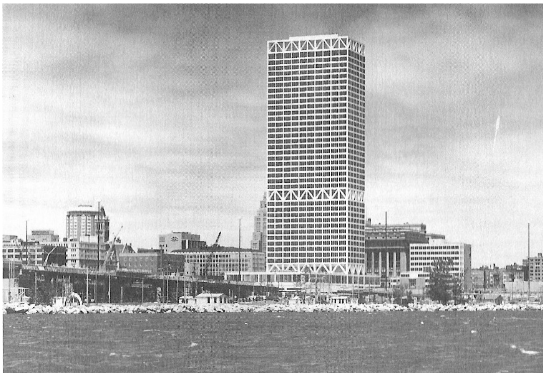
Graham and Khan considered the First Wisconsin Center's belt truss system worthy of bold expression. The 42-story building was completed in 1974. (Ezra Stoller © Esto.)
