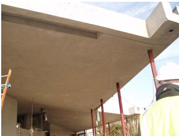
Exposed concrete ceiling. Note carefully designed formwork joints.
